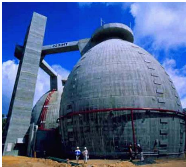
Figure 3. Sludge digesters at Woodmans Point sewage treatment plant, Western Australia. (Photo: Sustainable Energy Development Office Western Australia).
